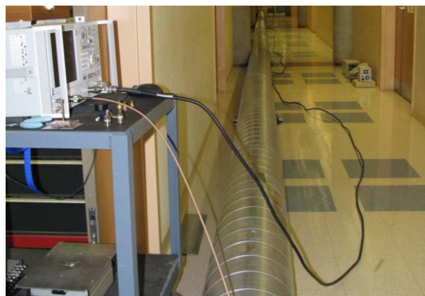
Fig. 5. Experimental setup for duct channel testing.
