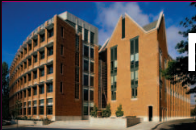
STEVEN'S ROAD-BENTON LANE ENTRANCE TO THE MICROSOFT ATRIUM AND THE NEW PAUL ALLEN CENTER (LEFT) AND EE BUILDING (RIGHT). THE SECOND AND THIRD FLOOR WINDOWS AND MOST OF THE BRICKWORK ON THIS EASTERN END OF THE EE BUILDING WERE FINISHED, AS PART OF THE CONSTRUCTION.
